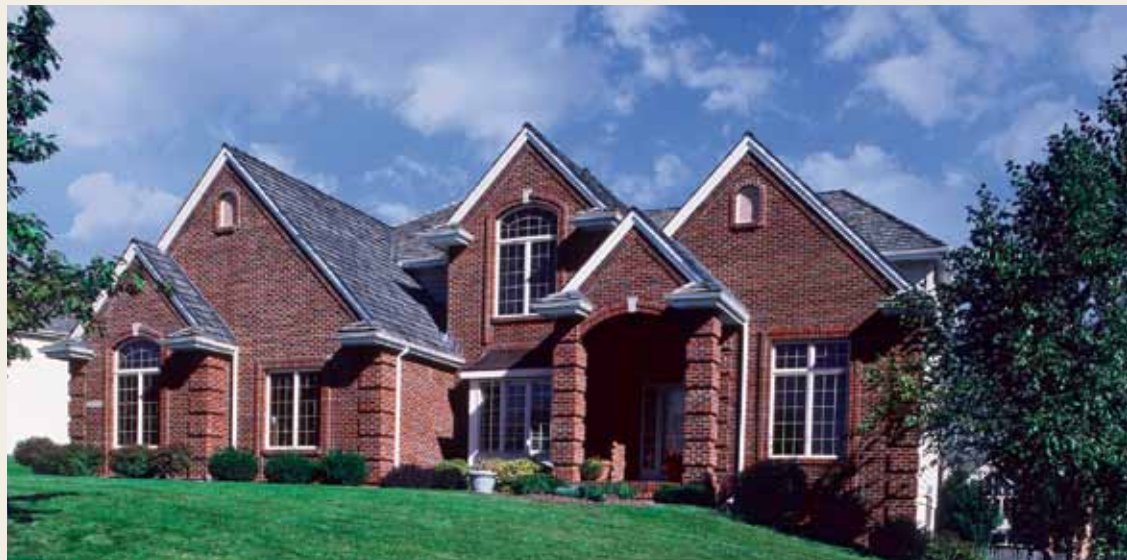
Private Residence – Lincoln, Nebraska Burgundy Sands; Heritage Texture
